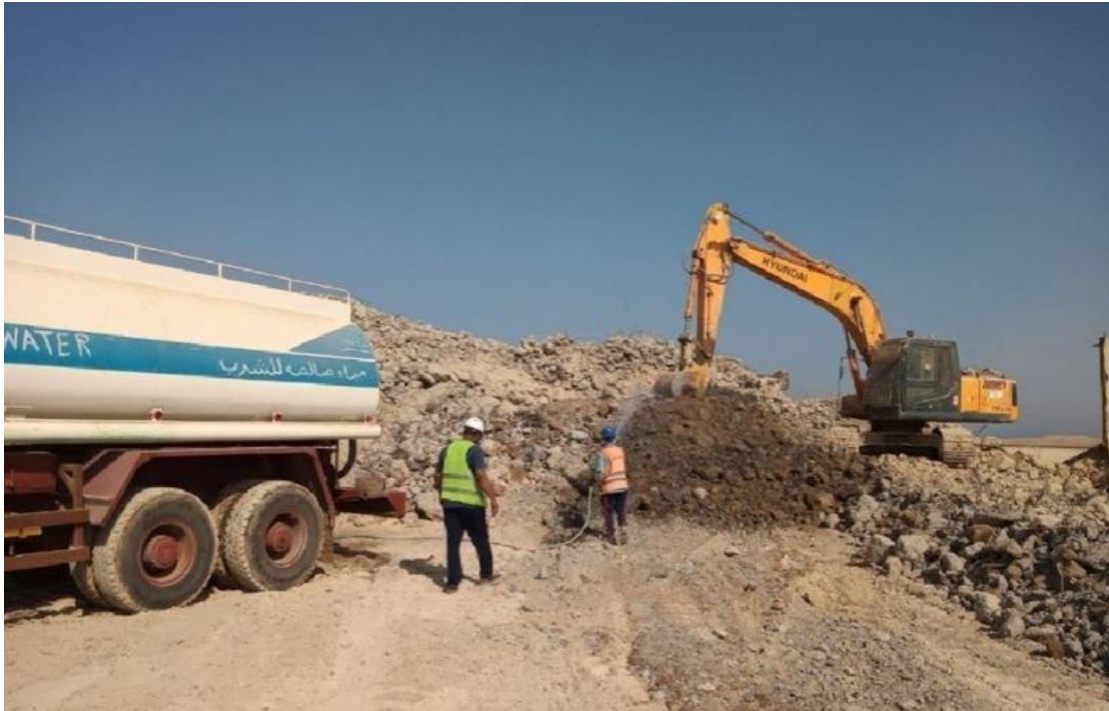
Figure 2,3. Stockpile wetting during loading activities.
