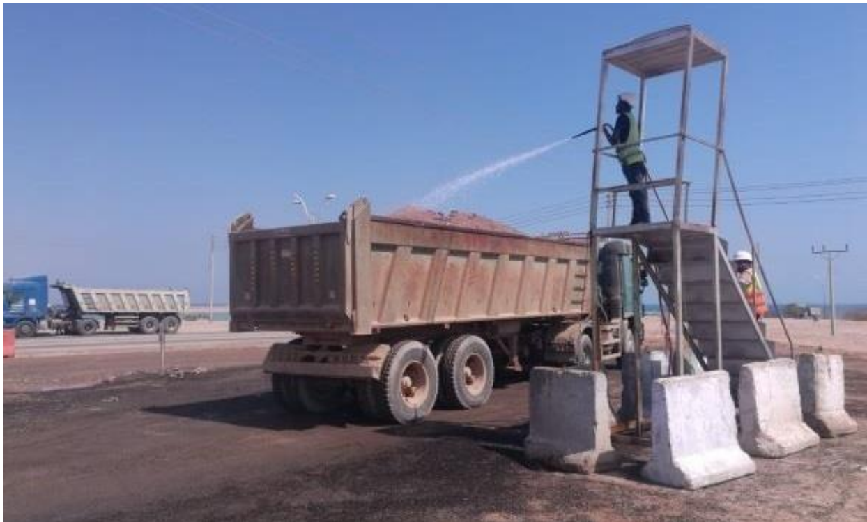
Figure 9. Wetting stations for wetting materials prior to tarping.
