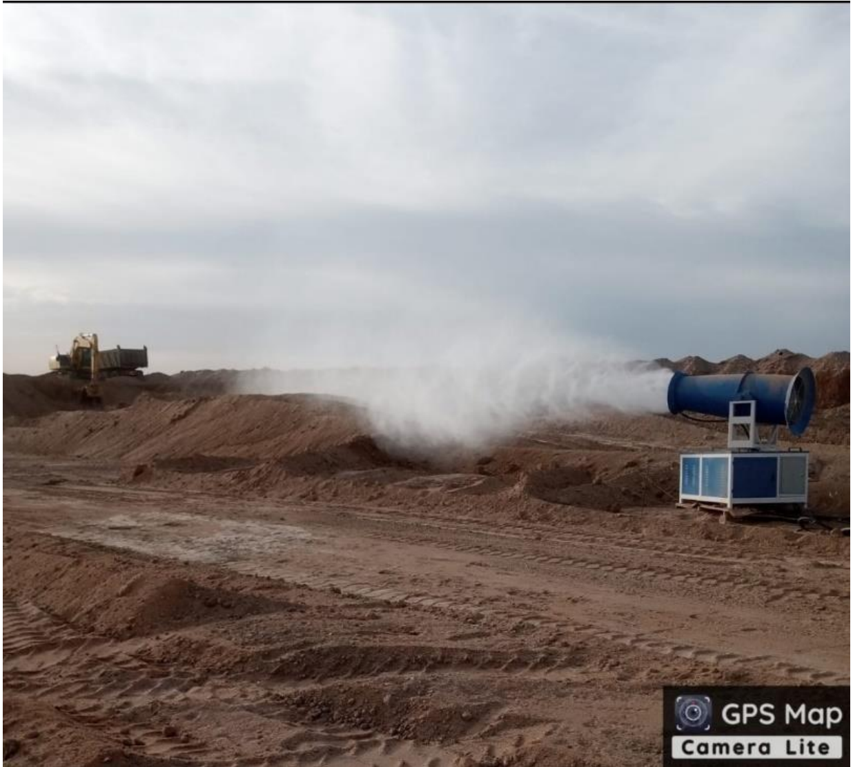
Figure 5. Water cannon misting stockpiles during loading activities (TSE not permitted for misting).
