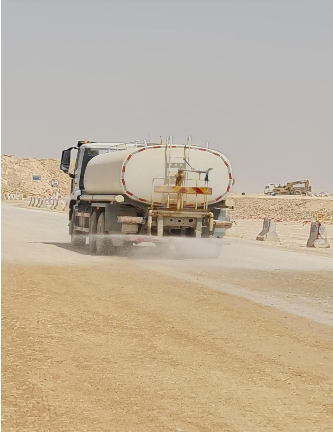
Figure 1. Road wetting by water truck.
