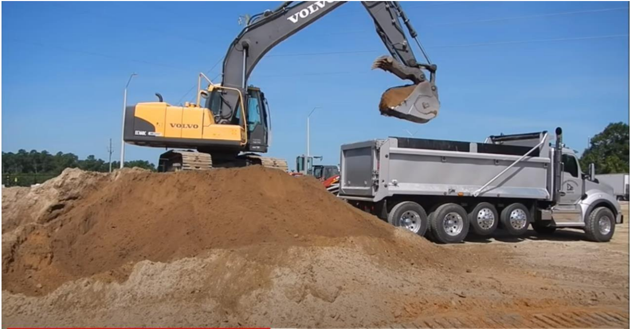
Figure 8. Loading materials at elevated platforms to minimize dust emissions by gently placing material rather than dropping from a height (Copyright – Google photo).
